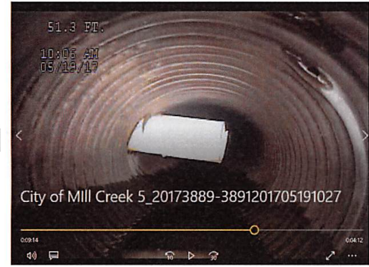
2. PVC pipe penetrating wall
